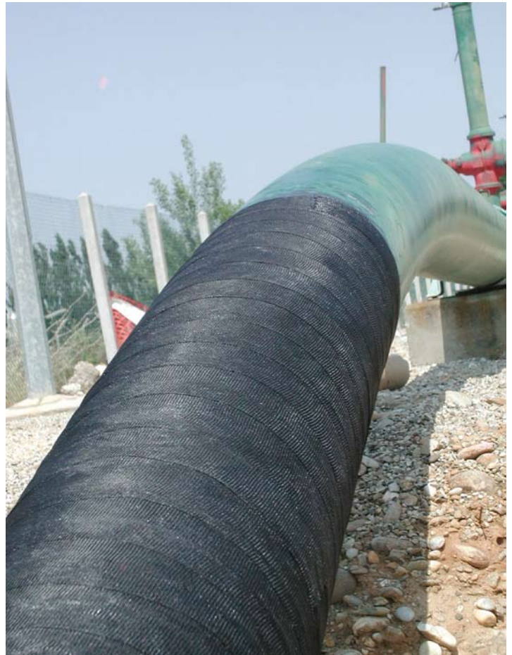
The "MC" in MC Outerwrap stands for "moisture cured." The materials in the wrap start to cure when they are exposed to the moisture in the air. Soon the wrap provides a very hard and tough outer coating.
