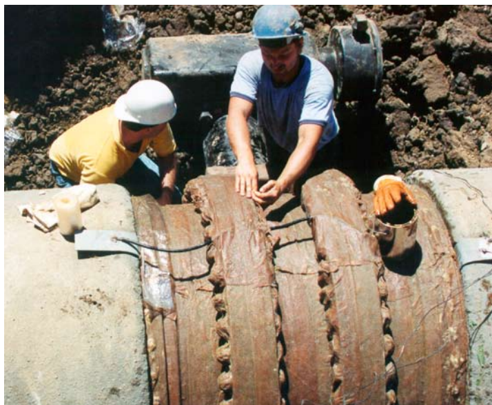
Trenton's #1 Wax-Tape is used in the water industry and conforms to AWWA Standard C217.
