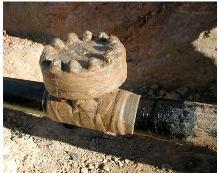
Trenton's #1 Wax-Tape protects irregularly shaped underground fittings and is compatible with cathodic protection.
