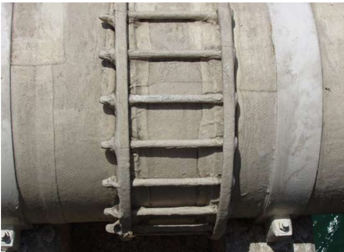
Wax-Tapes can outperform paint in many situations, lasting much longer and providing better mechanical protection.
