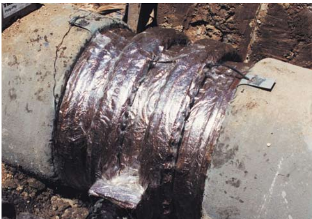
Poly-Ply is a multi-layer version of plastic wrap. It helps keep a separation between the tape and the soil.
