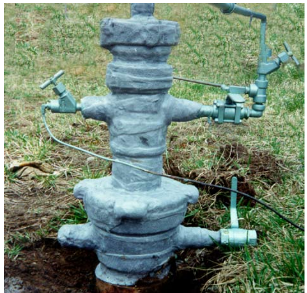
Trenton's #2A Wax-Tape completely conforms to irregular surfaces, such as this gas wellhead, and is unaffected by the elements.
