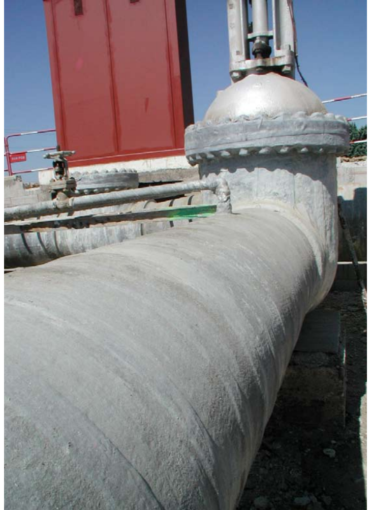
Many companies now use Trenton Wax-Tapes where they previously would have used paint.
