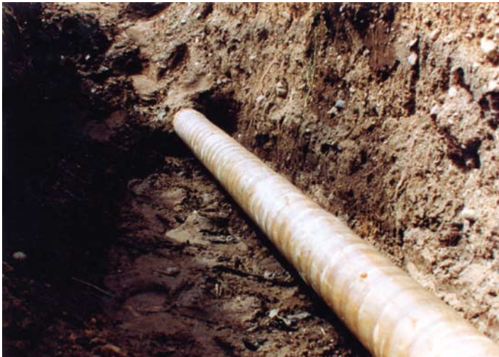
This is a section of 16" pipe reconditioned using #1 Wax-Tape and Glas-Wrap.
