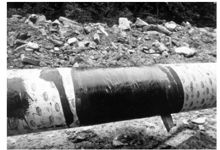
Finished application of Innercoat wax overwrapped with Guard-Wrap wrapper.
