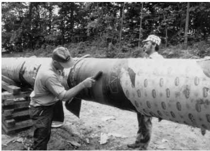
Pipe surface is wire brushed to remove loose scale, rust and dirt.
